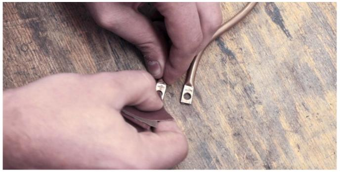
Fig. 51: Sanding contact surfaces
