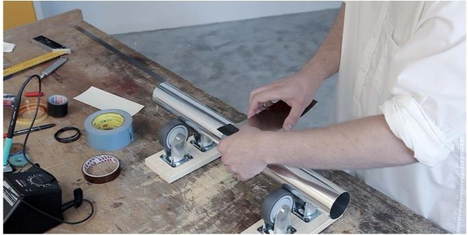
Fig. 31: Apply second Mu metal layer
