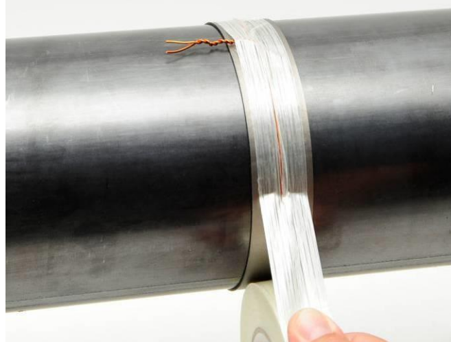
Fixed it with 3 layers mounting tape
